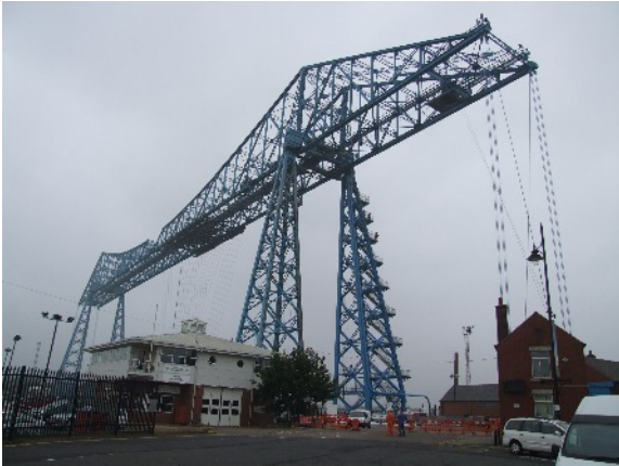
MIDDLESBROUGH TRANSPORTER BRIDGE
